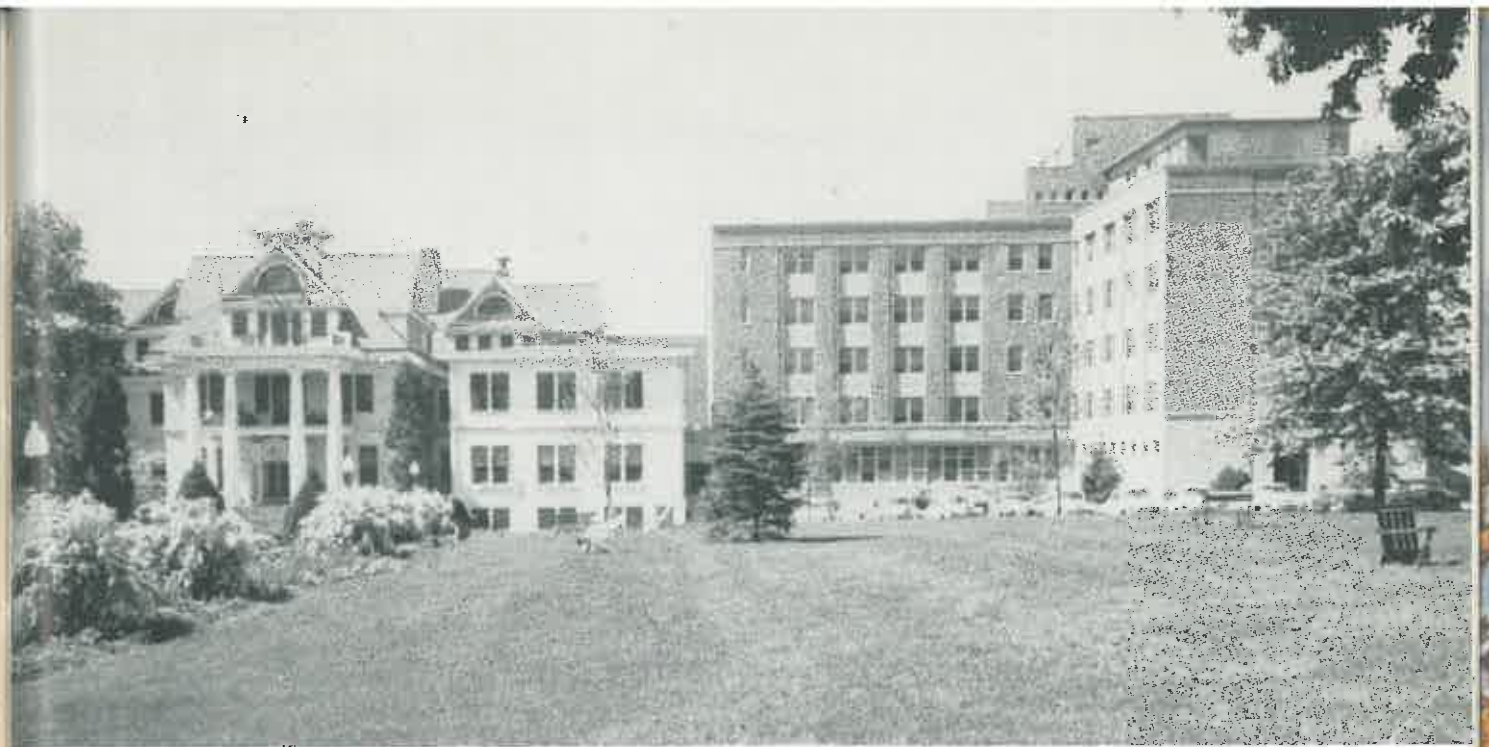
WASHINGTON SANITARIUM & HOSPITAL Takoma Park, Maryland
