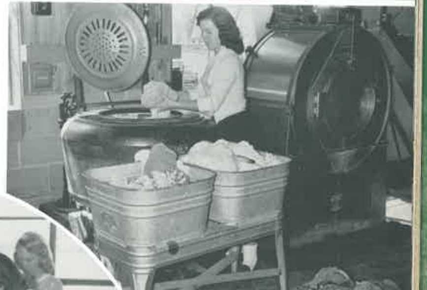
The laundry, a most important and efficient operation, is capably run by Mrs. Milliken. Peggy Viar is pulling clothes out of the extractor to be placed in the dryer.
