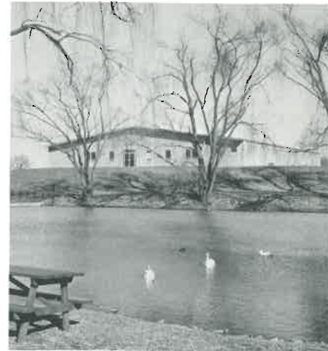
Newly Constructed Bindery
